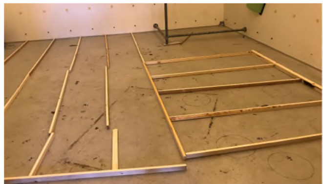
Spacers laid out before mounting of Acupanel
